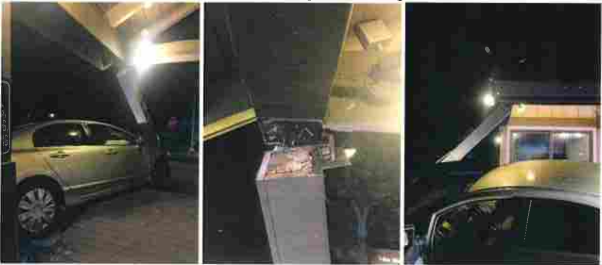
Exhibit 5 Site Photos of Damages to the Existing Guardhouse
