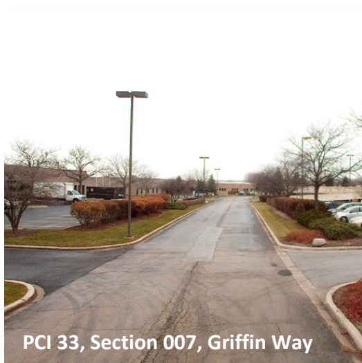
Figure 7. Sample pavement images with different PCI values.
