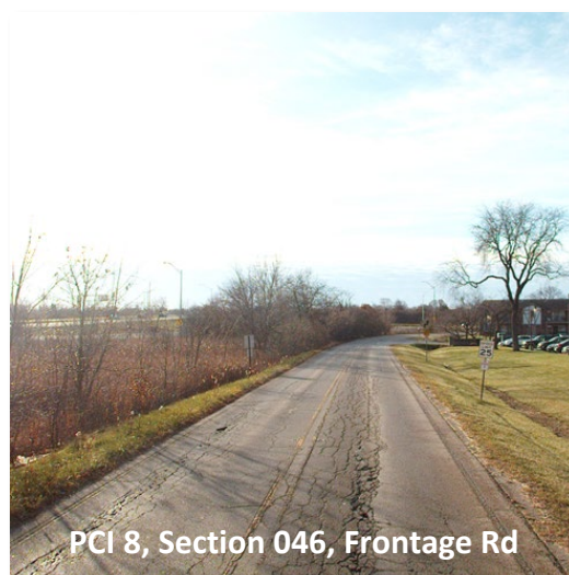
Figure 7. Sample pavement images with different PCI values.
