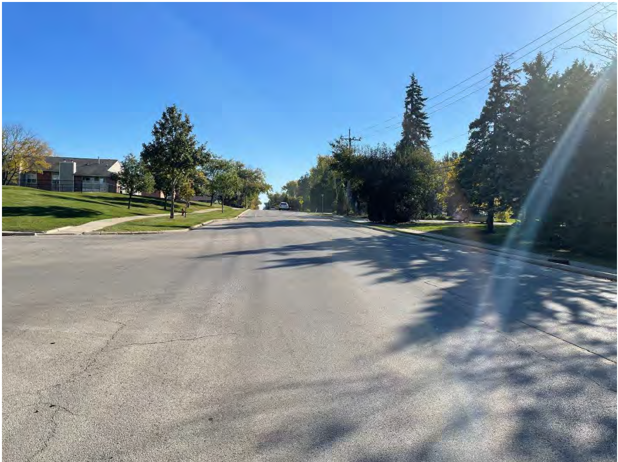
Image C: Vertical Curve on Clarendon Hills Road as Viewed from MacArthur Drive
